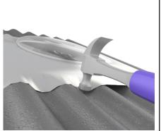
Using a hammer or rubber mallet, gently form the edges of the tray to match the roof profile.
