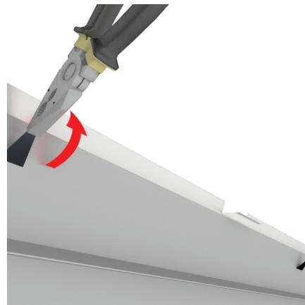
Attach flexi shaft to aluminium shroud by piercing the tabs through the shaft and folding upward with pliers.
