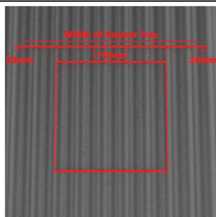
From out on roof, use the inside throat as a template for cutout of skylight. Extend the top edge up 70mm. Mark a line full width of soaker tray, plus 10-15mm each side.
