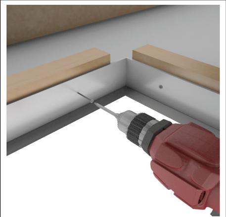
Secure the ceiling frame to ceiling by driving screws through ceiling frame collar into joists/trusses if available.
