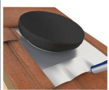
Seal under bottom and side edges with silicon.
