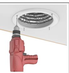
Using cordless drill, fix ceiling ring to ceiling with screws provided.
