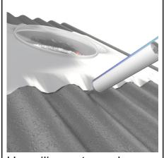
Use silicone to seal under edges of the top and bottom of the tray to roof sheeting.
