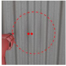
Using a drill, mark the edge of where the dome will be located on the roof sheeting.
